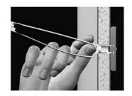
Place thumb between straps at ceiling and push thumb side to side, snapping off straps level with flange of cap.
